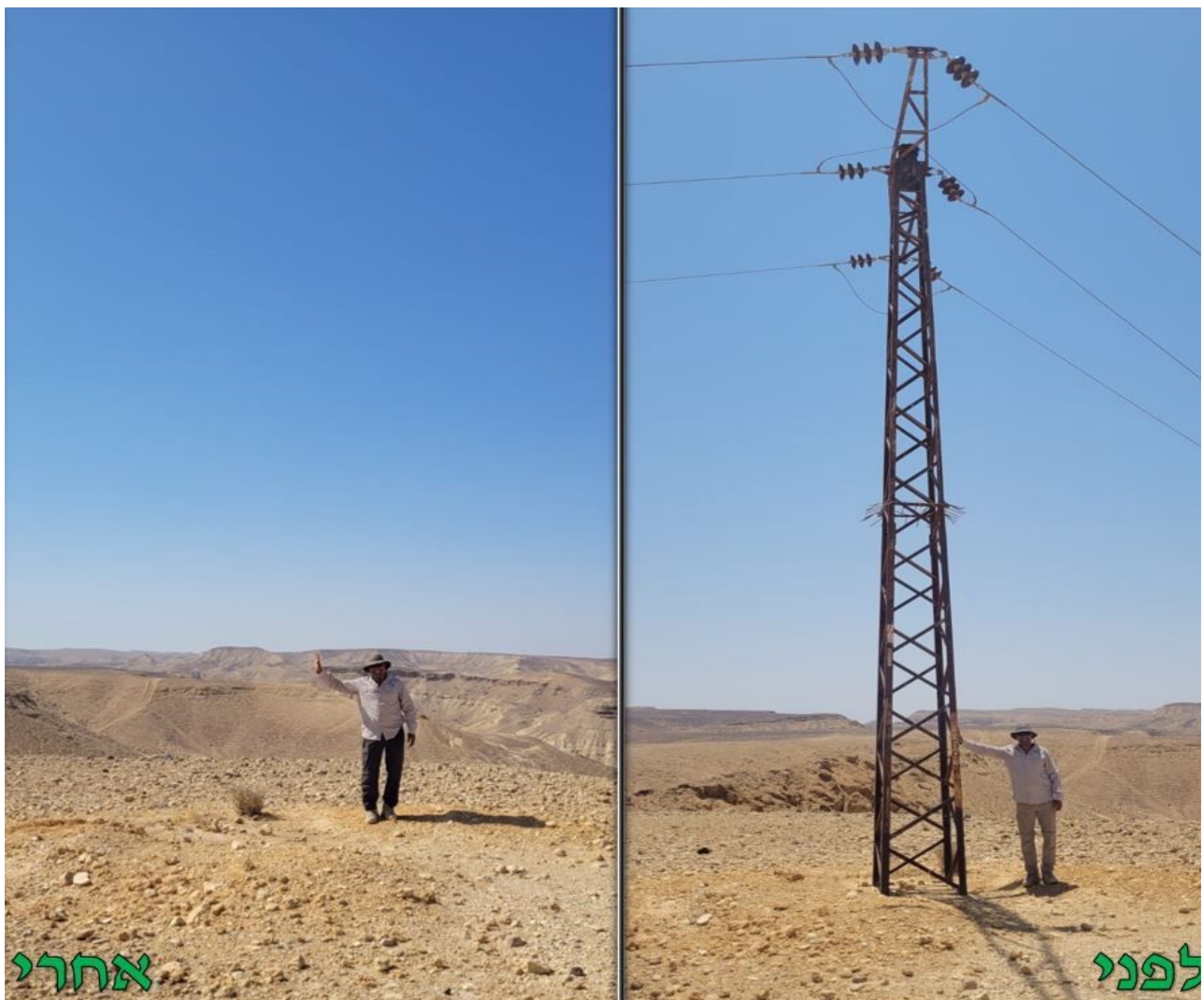
Dismantling of the power line in the Dimona region, before and after; as shown, full ecological and landscape restoration of the area of the poles and the worksite were performed.
