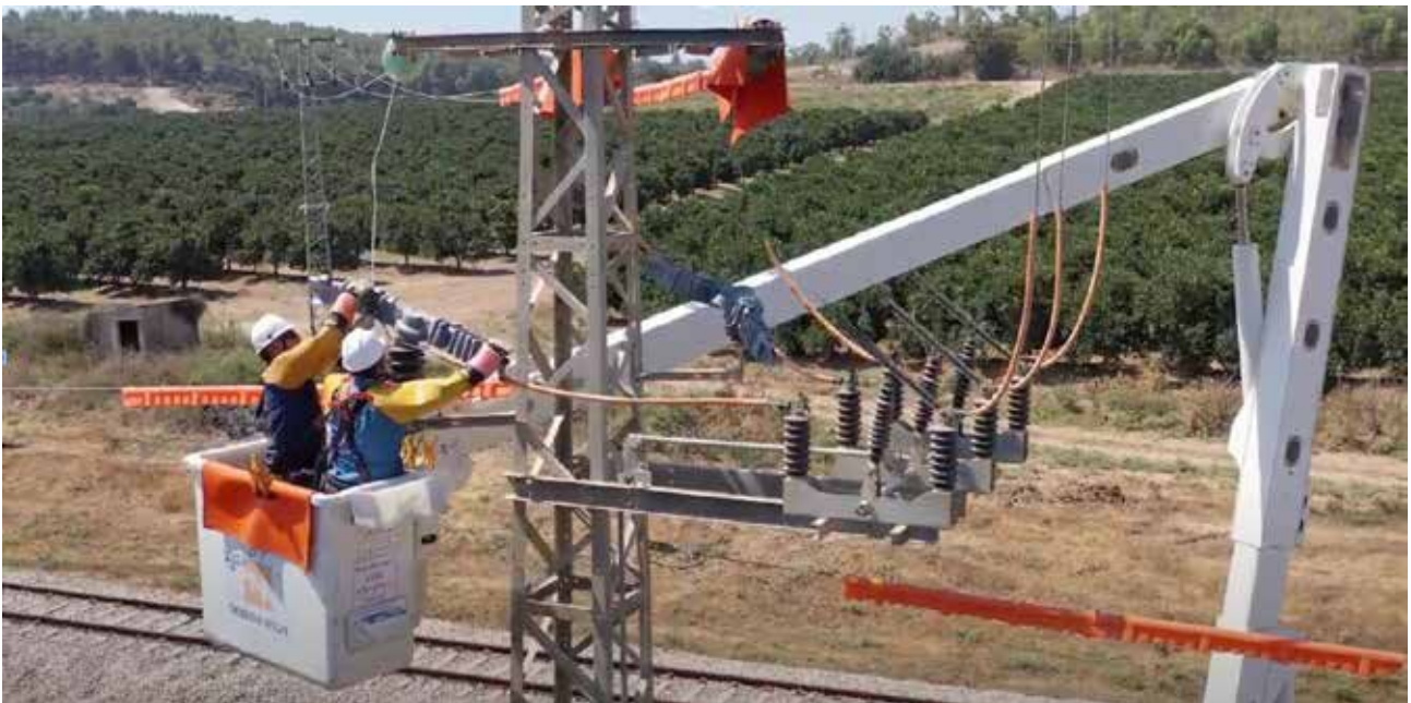
IEC employees safeguarding a high-voltage pole to prevent the electrocution of birds of prey; Tal Shachar region.
